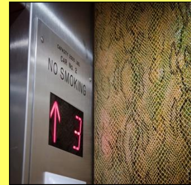
Lifts (for those buildings which go below ground level)
